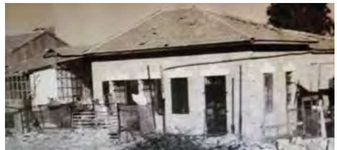
In this building the first home for abandoned babies and School for Nurses opened in Jerusalem's Sha'arei Hesed district.
